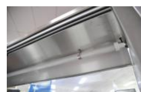
Top mounted fluorescent lighting
