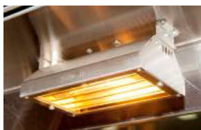
Quartz infrared overhead heat lamps
